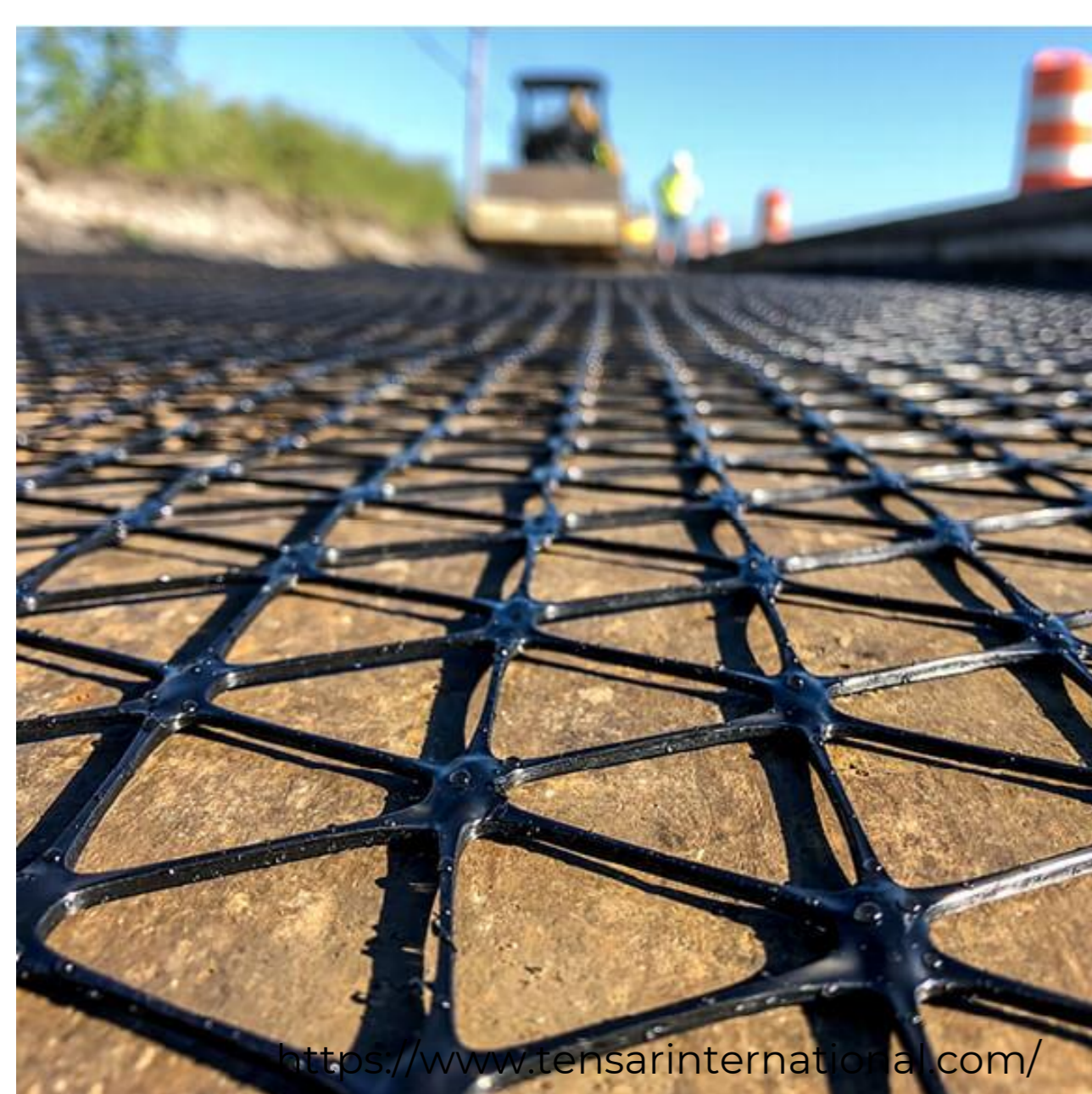
Figure – Geogrid for pavement reinforcement
